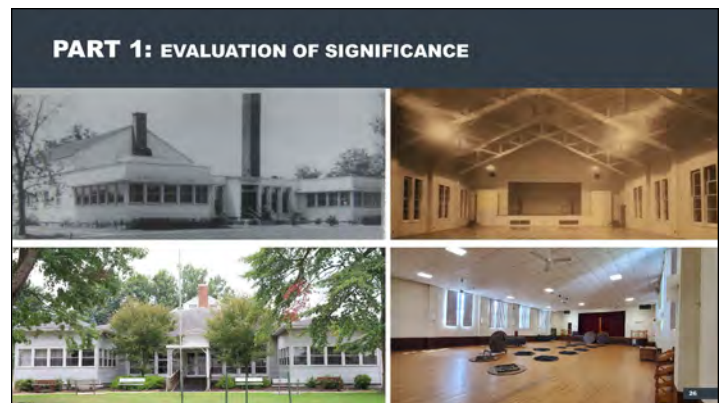
Historic images of this USO building identified changes to the exterior roof structure and interior ceiling of the main room, which can inform future restoration efforts.
